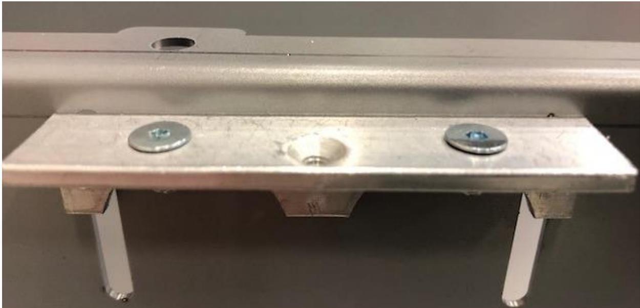
**\*A). Typical installation using the mounting brackets.**
